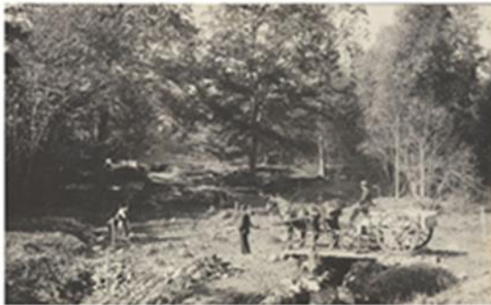
Boston Parks Commission. Road construction, Valley Road at Bussey Brook, 1892
