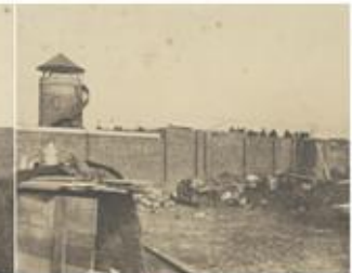
A8 - Construction. Upper garden wall, inside garden
