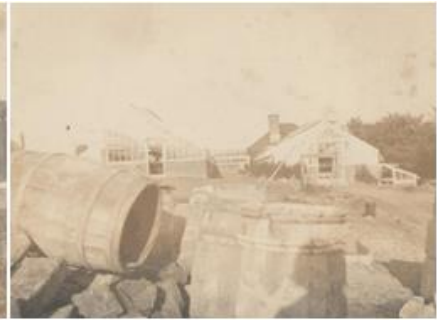
B9 – Construction. Upper garden major axis (see A nos 9,6,3,2) (pg. 99 in Spirit of the Garden)
