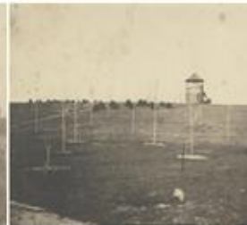
A7 - Hill site showing existing tower (Greenhouses lay to the right.)
