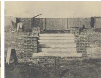
D8 – Construction (see No 5)
