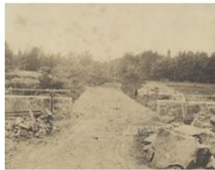
E5 – Construction. New entrance toward swamp (Trees at right same as A1)
