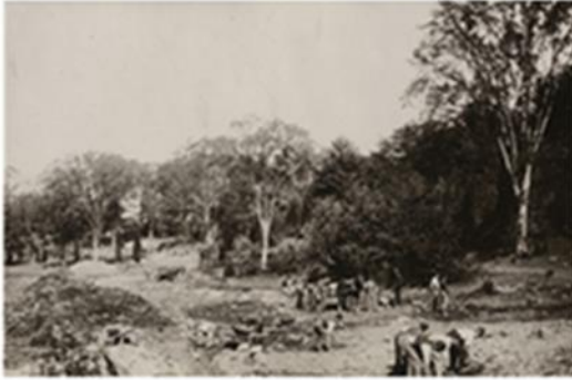
Boston Parks Commission. Road construction, Hemlock Hill Road, 1889
