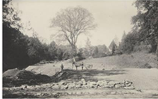
Boston Parks Commission. Road construction, Valley Road at South Street, 1891
