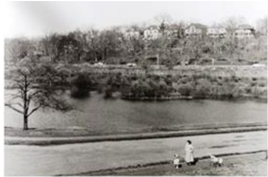
Flooding, Dawson Pond, 1958
