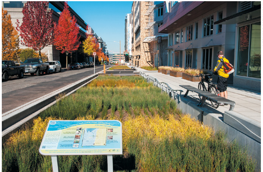
Seattle's “Swale on Yale” offers attractive planting beds that also serve to filter runoff.
