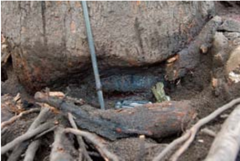
Figure 2. With part of a stem girdling root removed, the compression to the tree's trunk is evident.
