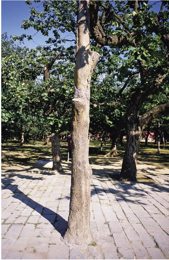
18: Tree support, concrete. Ming Tombs, Dingling, China, 2005.
